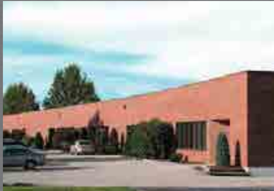
Turret Manufacturing Facility Chesterfield, MO, USA
